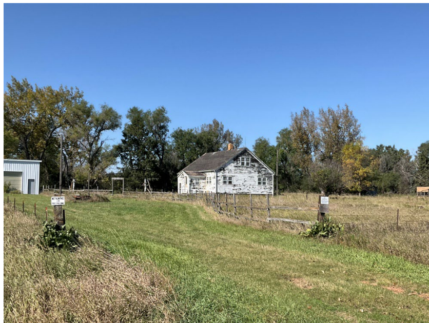
Photo 18: 32MOX842 (MER-494), view facing west toward the house
