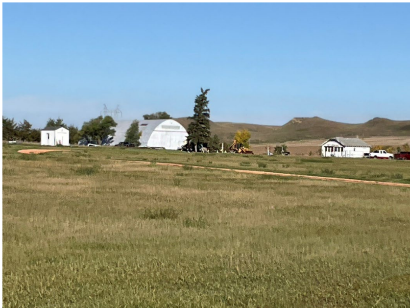
Photo 24: 32MOX845 (MER-509), view northwest of Quonset workshop and garage
