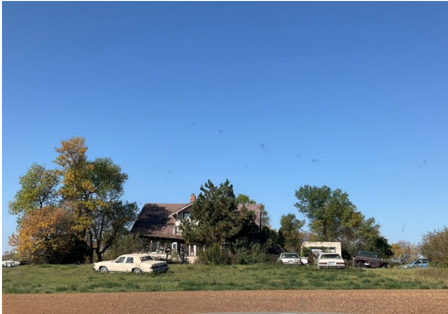
Photo 5: Site overview looking west, 32MOX832 (MER-444)
