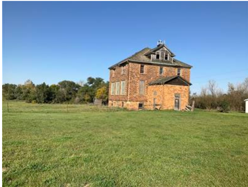
Photo 2: East facade and south elevation of the St. Clements school
