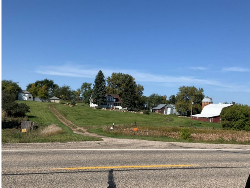
Photo 13: Overview looking west, 32MOX840 (MER-460)
